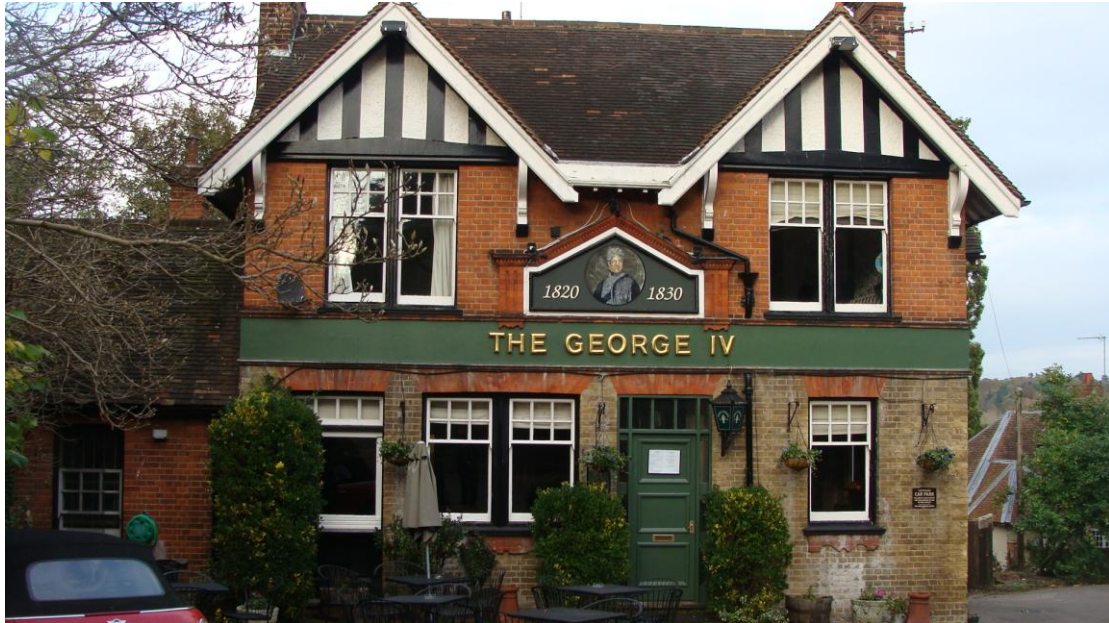
Picture 12. The George IV PH. A late 19th/early 20th century building of quality with many architectural features worthy of preservation through normal development control.
