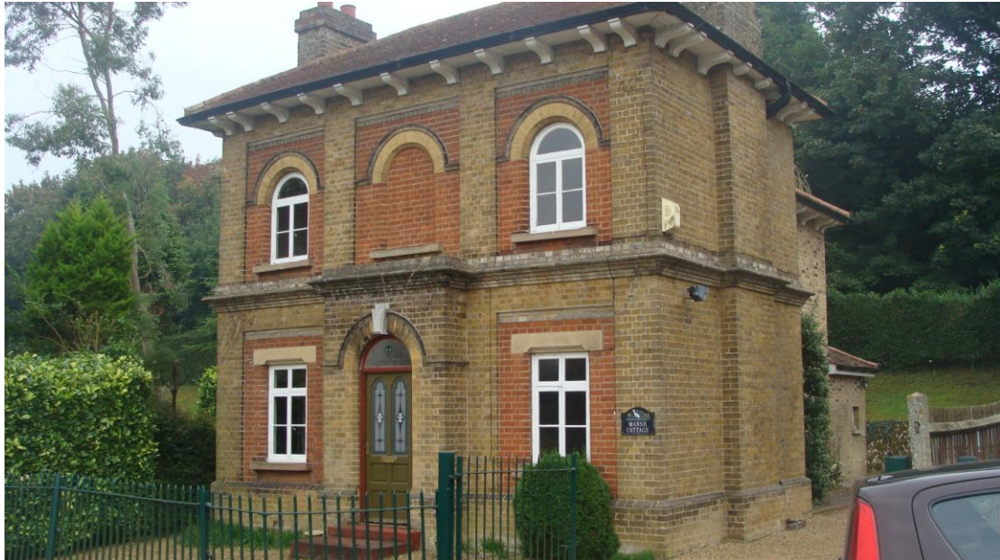
Picture 10. Marsh Cottage, former engineers house associated with the adjacent pumping station.
